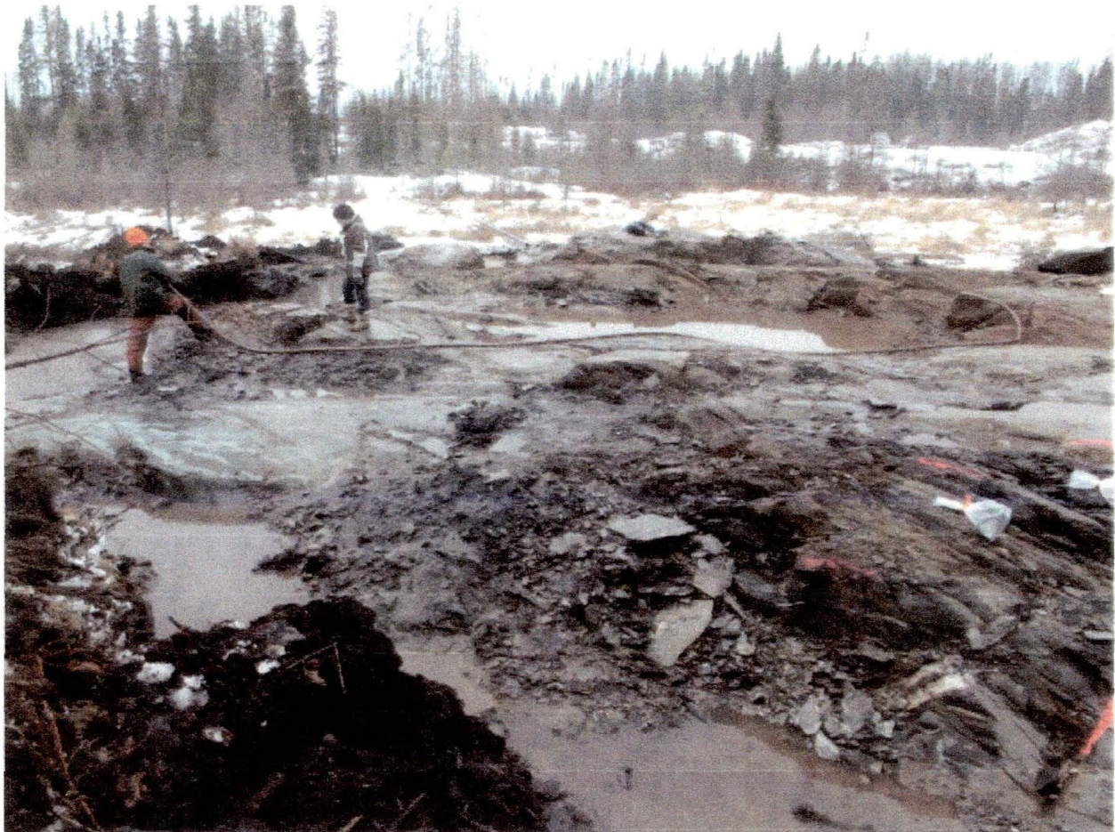
Main Shear South - Trenching December 2011
