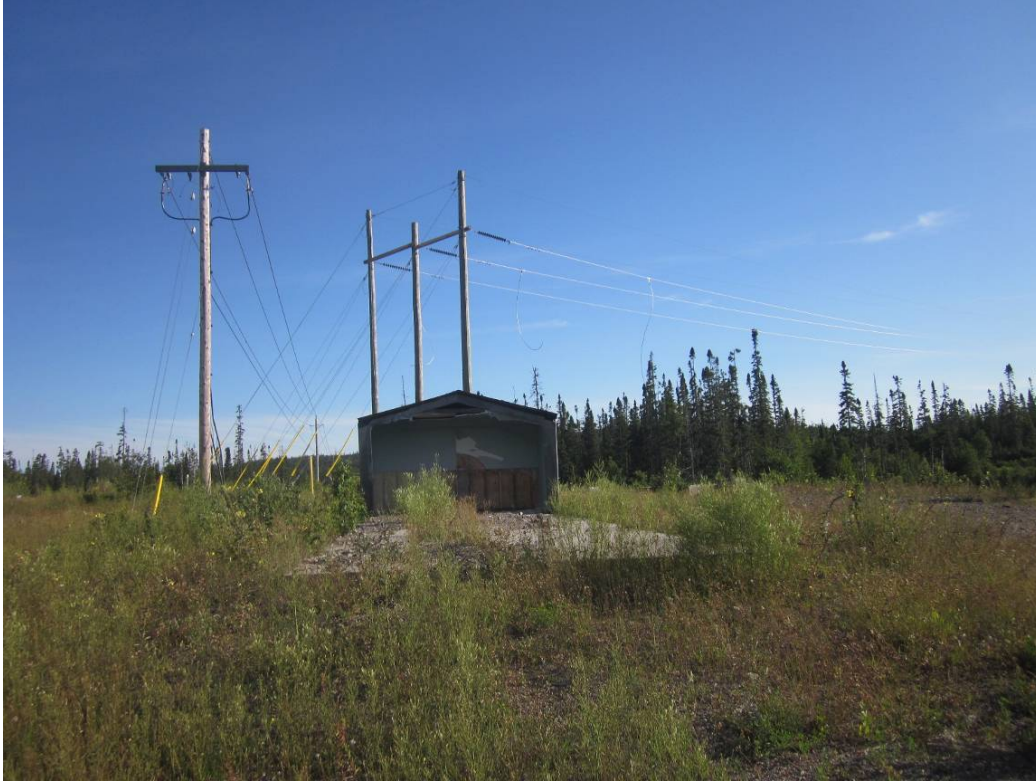
Figure 20: Surface of the C18 Anomaly and the Old Mine Infrastructure for Pick Lake Deposit
