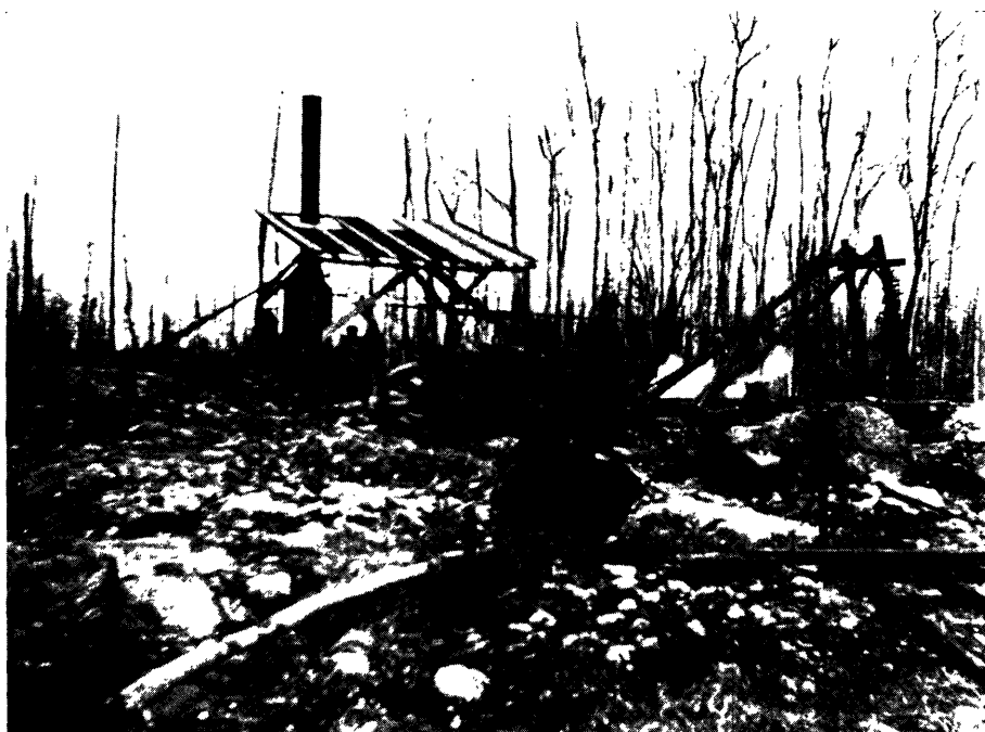
Small steam plant on McRae property.
