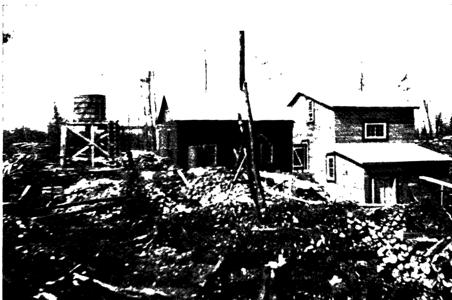
Power plant and mill at Miller-Independence property.
