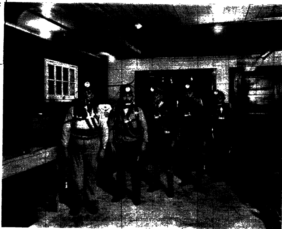
Rescue team wearing McCaa two-hour breathing apparatus, Timmins mine rescue station.
