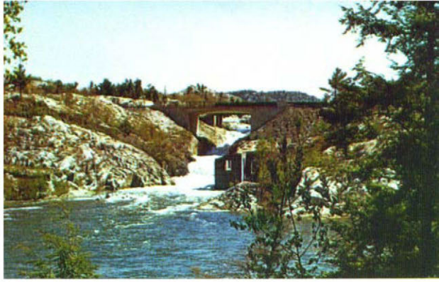
Photo 71. Whitefish Falls and the road bridge carrying Highway 68.
