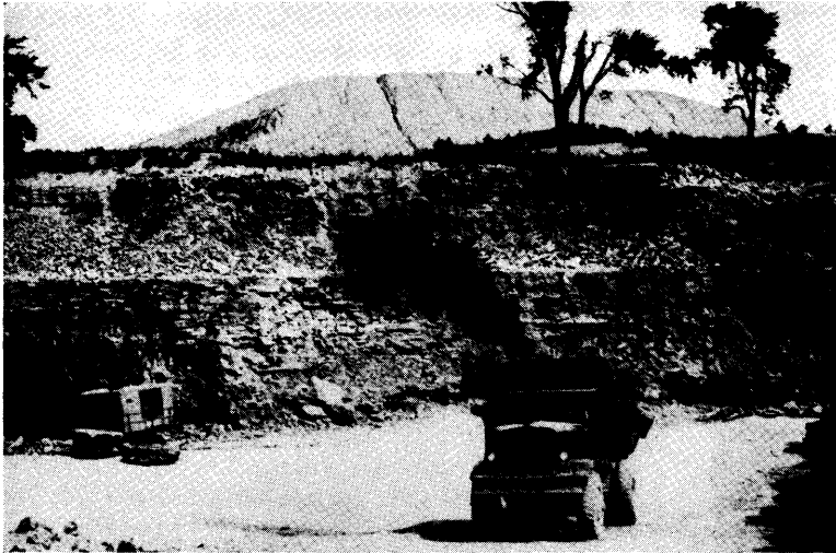
Eramosa dolomite of the Lockport formation at the Vinemount quarry of Armstrong Brothers Company Limited. A Euclid truck is seen in the foreground.
