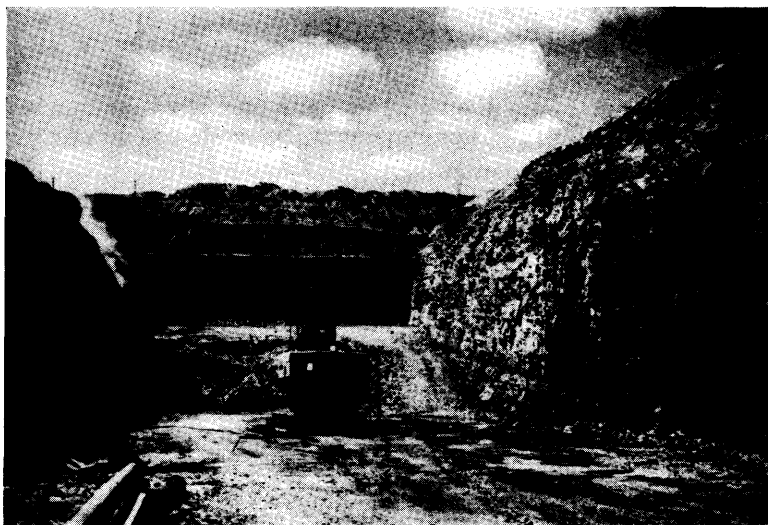
Canada Cement Company Limited quarries 100 feet of high-calcium Detroit River limestone at their Woodstock plant; 70-80 feet of overburden is stripped. The photo shows the Joy Heavyweight Champion rotary drill in action.
