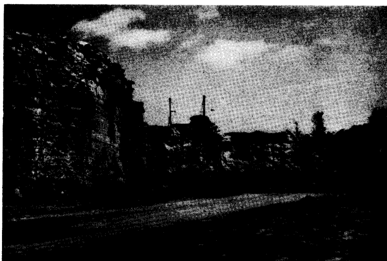
The quarry of Ottawa Valley Crushed Stone Limited, near Ottawa, exposes 70 feet of Middle and Upper Black River limestone. Churn drills may be seen operating in the background.
