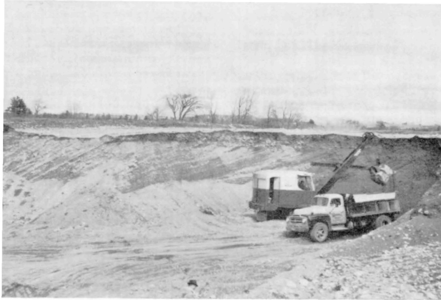
Iroquois beach deposit operated by Consolidated Sand and Gravel, Pickering.
