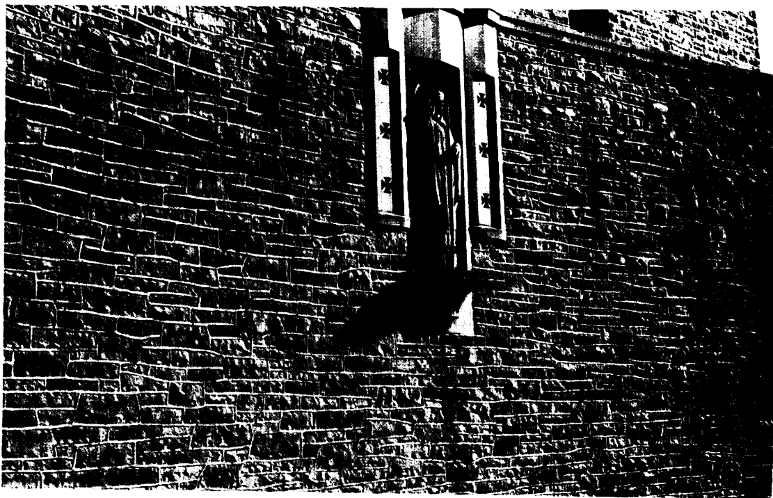
Split faced Medina (Credit Valley) sandstone rubble used in St. Augustine of Canterbury Church, Bayview Avenue, Toronto.
