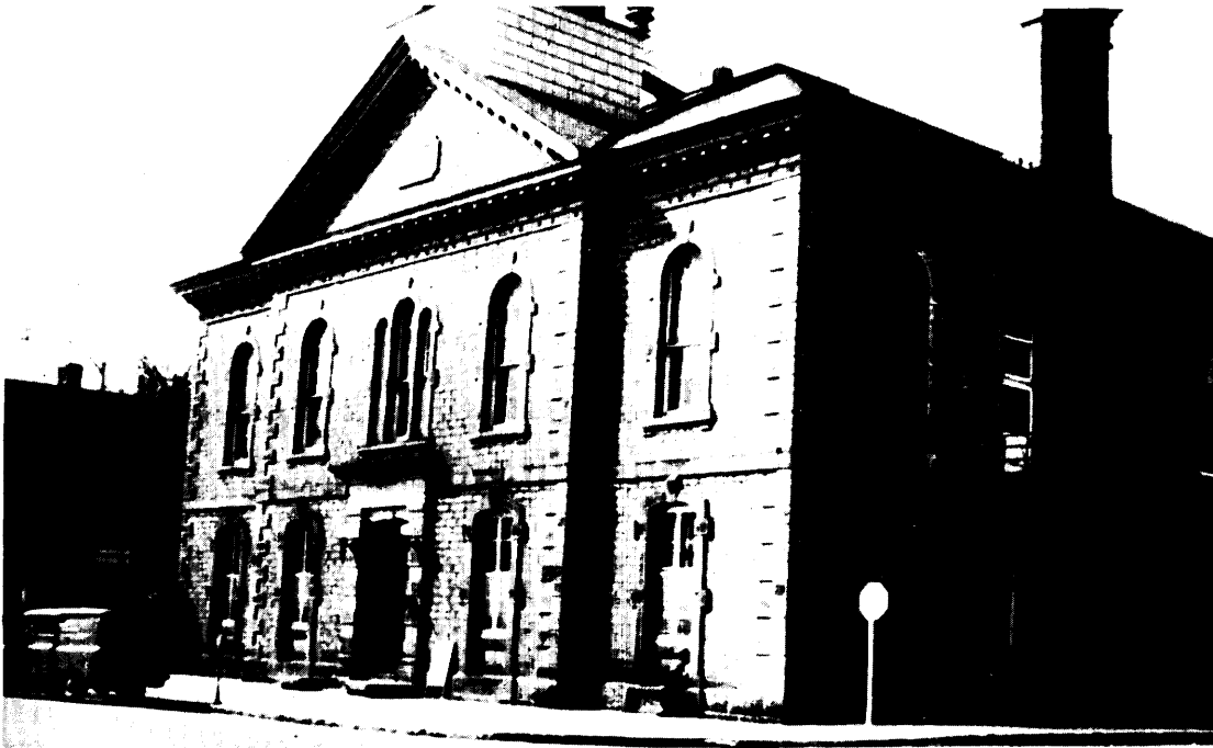
Perth town hall erected in 1863 using local grey and purple Potsdam sandstone.
