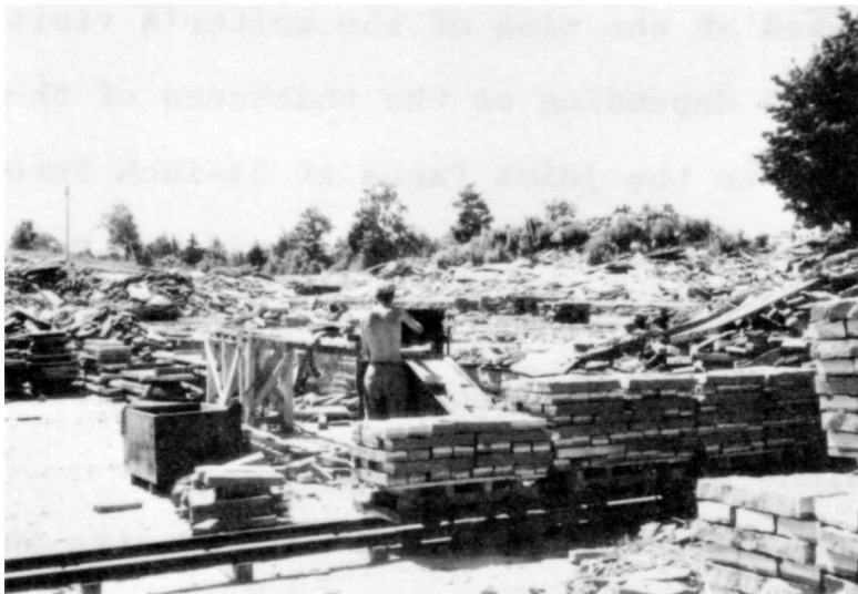
Ashlar split by guillotine is loaded on pallets for shipping at Ebel Quarries, Wiarnton.
