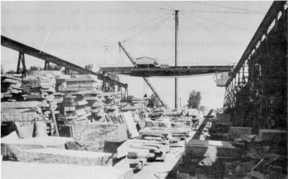
Stone yard at Queenston Quarries showing overhead crane.
