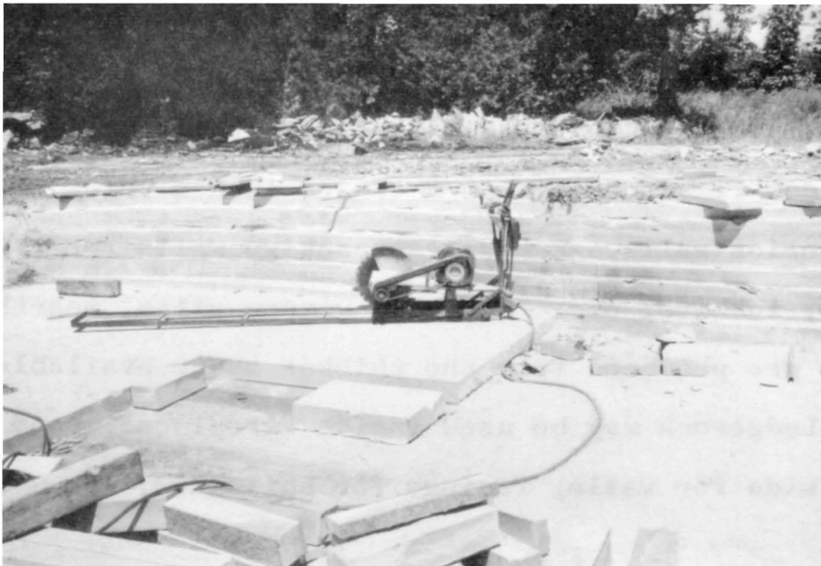
Portable diamond saw used for cutting Eramosa dolomite near Wiarton.
