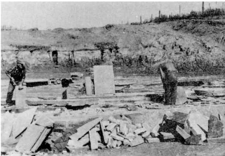
Trimming flagstone at Rice & McHarg quarry, Limehouse.
