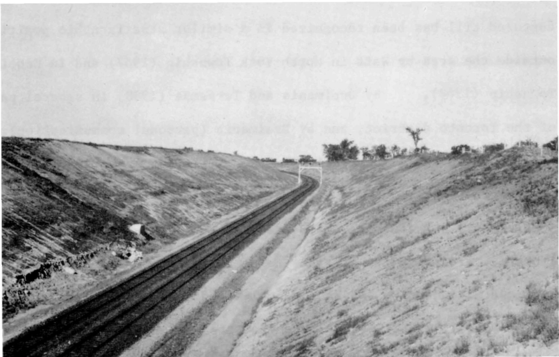
Photo 4. Canadian National Railways Bypass cut in thick Leaside Till west of Yonge Street.
