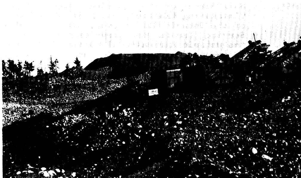
Caswell gravel pit, lot 5, concession V, Henwood township: portable crushing and screening plant.
