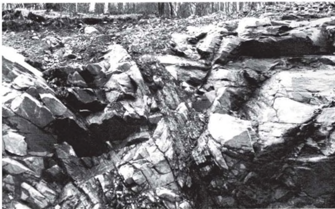
Photo 27 The Brewer Lake fault, mile 32.0.
