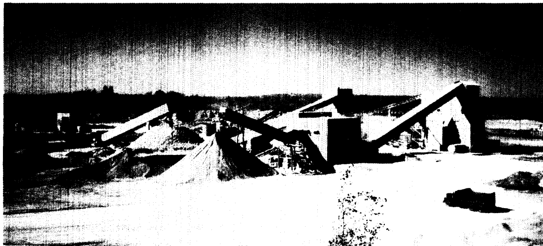
Photo H-5-2. UHTHOFF QUARRY PROCESSING PLANT, SHOWING RAIL LOAD-OUT (RIGHT).
