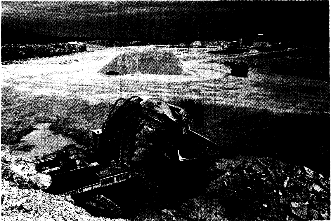
Photo CB-4-1. O & K (17 YD.) HYDRAULIC EX- CAVATOR LOAD- ING 85-TON TEREX TRUCK AT THE WORKING FACE OF THE MILTON (DUFFERIN) QUARRY; PROC- ESSING FACIL- ITY IN BACK- GROUND (LOOK- ING NORTH- EAST).
