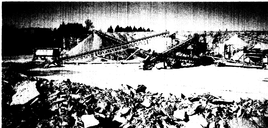
Photo H-8-1. PRIMARY FEED HOPPER AND PORT- ABLE CEDARAPIDS IMPACTOR CRUSHER; GAMEBRIDGE QUARRY.
