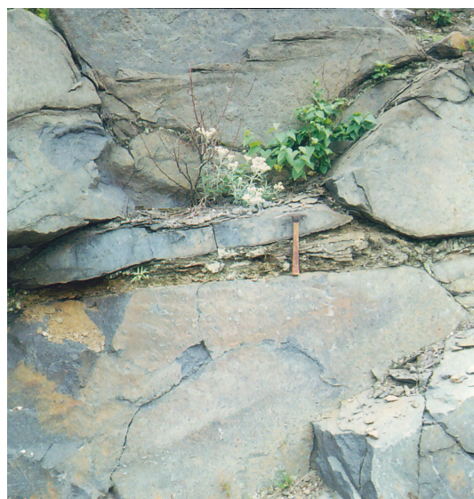
Photo S11. Gertrude Fault.
