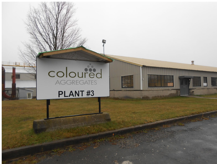
Photo 4. Coloured Aggregates plant entrance and office area, Marmora, Ontario.
