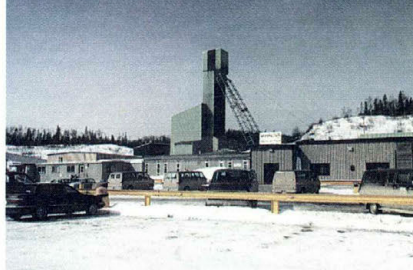
PHOTO 67: The tall building at Winston Lake Mine is the headframe. It stands over the mine shaft, and houses the hoisting equipment for the "cages" and "skips" used to move workers, supplies, waste rock, and ore.
